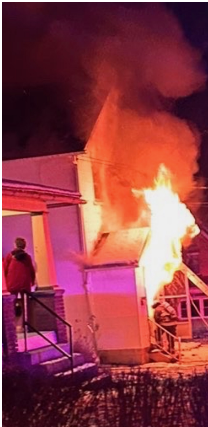
Shown above is Sharon Fire Department Captain Kevin McMahon preparing to make entry during a residential structure fire at 334 Prospect Street in Sharon on December 4, 2025, after crews were advised of possible occupant entrapment.
